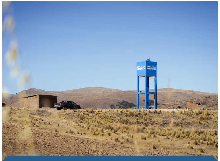
The elevated water storage tank you built
