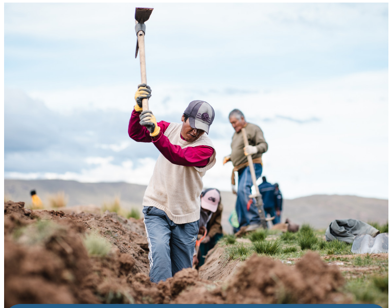
Residents digging trenches for the pipe network
